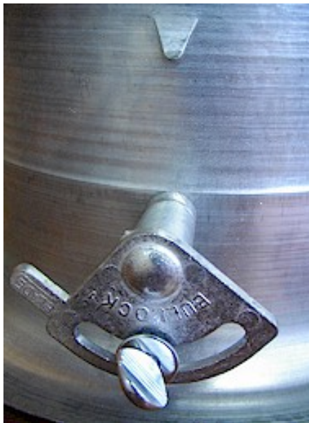
Raised die cast quadrant and duct retaining lance
